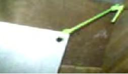
The plate is positioned between 3 and 3.5 metres (10 to 12 feet) above the ground and the attachment to the plate is also heavy-duty 8 swg cable:
