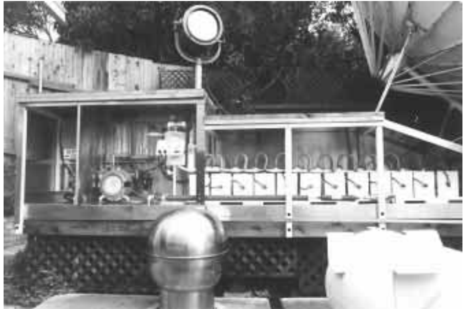
Above: An overview of the electrolyzer system. The power supplies and electrical controls are on the far left. Purification equipment is to the right of the power controls. The electrolyte reservoir and hydrogen and oxygen float valves with pressure gauges are to the right of the purification equipment. Twelve electrolyzer cells are shown on the far right. A feedwater purification system is just below the twelve electrolyzer cells. The caustic electrolyte storage tank is on the ground below the float valves.
